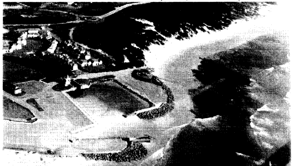
Figure 1 Longshore sediment transport problems at a harbour (photo taken by D Phelp along the Eastern Cape coastline on 28 September 2000)
