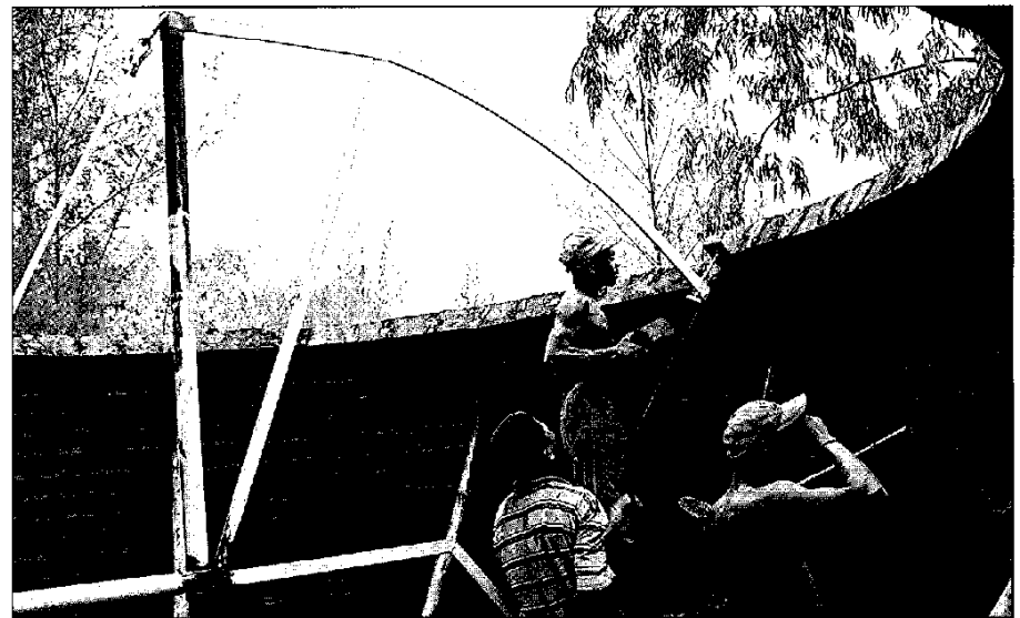
Figure 7 Guiding template to construct wall
