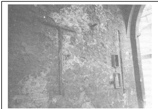
Built into the walls of the local congregation building (this one is the town hall of Laon) might be rectangles to gauge the size of bricks, others to measure roof tiles; lengths of metal to measure cloth or timber, and so on. It was the obligation of local officials to maintain fairness. In return they of course were entitled to extract a small fee.
